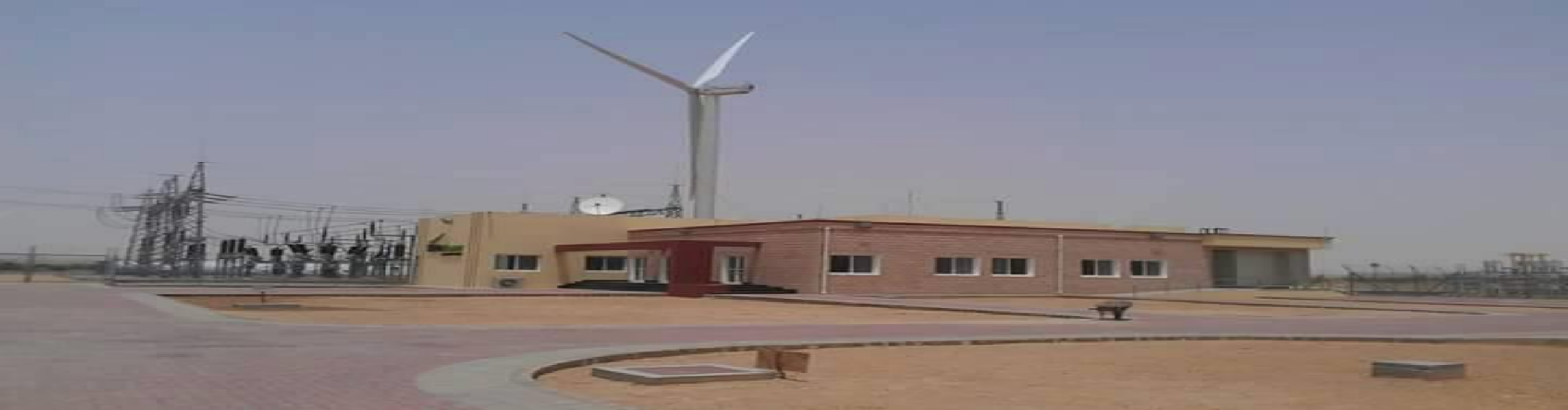
50 MW Yunus Energy Ltd Wind Power Project, Jhimpir, Thatta, Sindh Work Completed Achieved Commercial Operations Date
